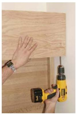
**Step 11**Concealing the guide rail screws with the wood buttons provides the final touch. If you are concerned about them working out, a dab of glue will prevent that from happening.
