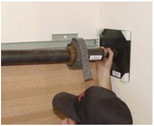
Place the short metal curtain slats in the collar notches and attach them using the 3/4" bolts provided.
