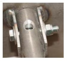
Before going any further – double check that the shaft bolt has been secured in place with the flat washer and capture nut.
